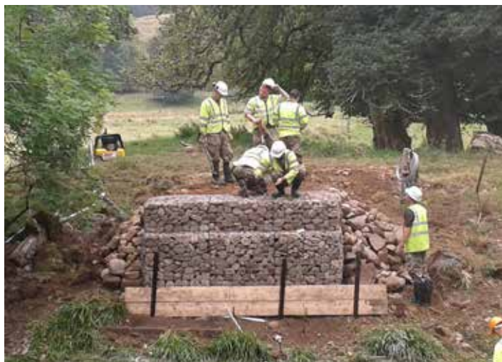
Building bridge abutments for the Orienteering World Championships
