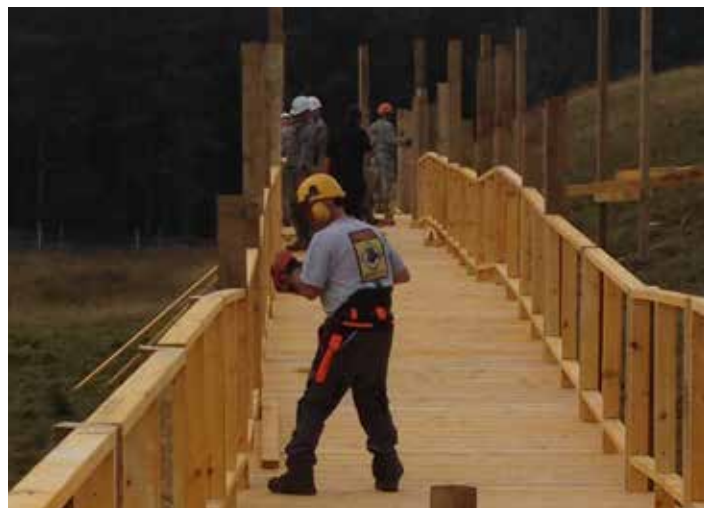
Constructing an elevated walkway at the Highland Wildlife Park
