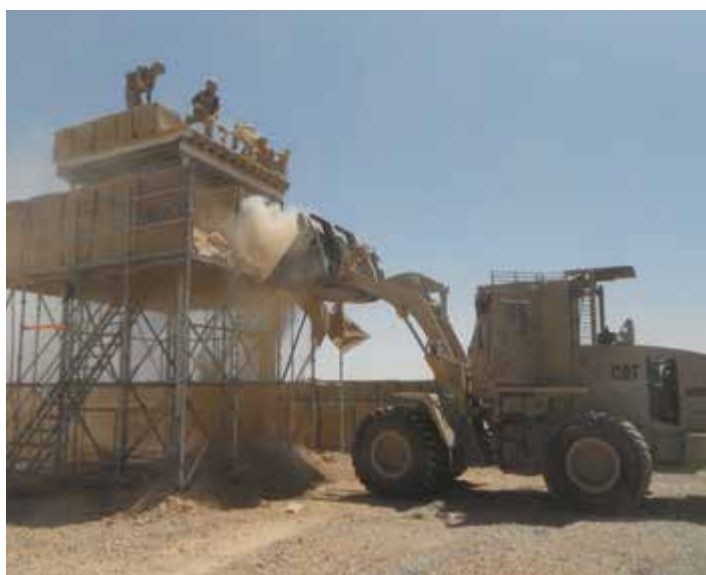
Deconstruction task using Armoured Plant in Afghanistan
