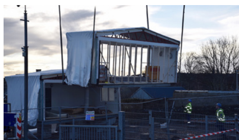
One of the modules being lifted into place and (right) the old cadet hut.
