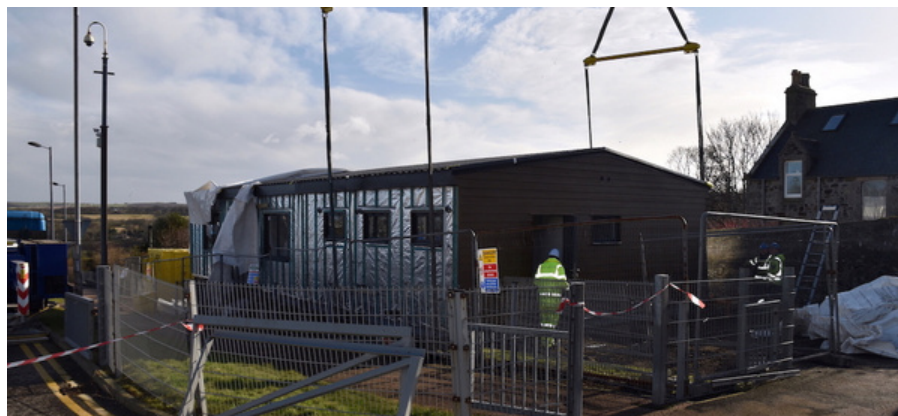
The new building arrived on site in five prefabricated sections.
