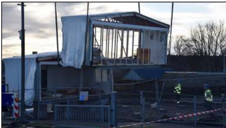
February 2022 – A section of the modular hut at Banff is lowered in.
