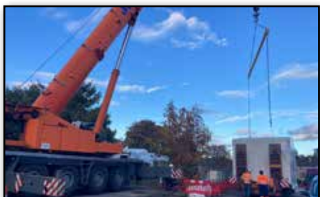
The sections arrived by lorry before being removed by crane and moved into place.
