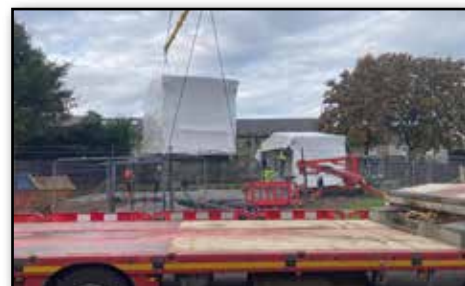
The sections arrived by lorry before being removed by crane and moved into place.
