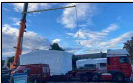
The sections arrived by lorry before being removed by crane and moved into place.
