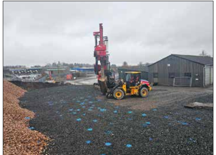
February 2024 – 350 piles were driven into the ground at the Dunfermline Army Reserve Centre site.
