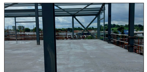
Two views of the frame of the new building and (right) the upper floor with its freshly-poured and levelled sub-floor.
