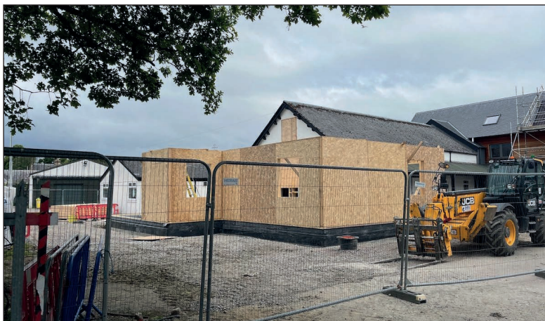
Some of the earlier works (above, and right) that saw the installation of the flat pack extension walls.
