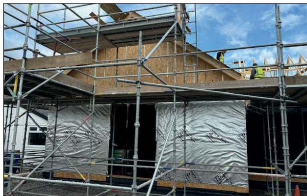
The latest images from Dingwall show the extension reaching the stage of being wind and watertight.
